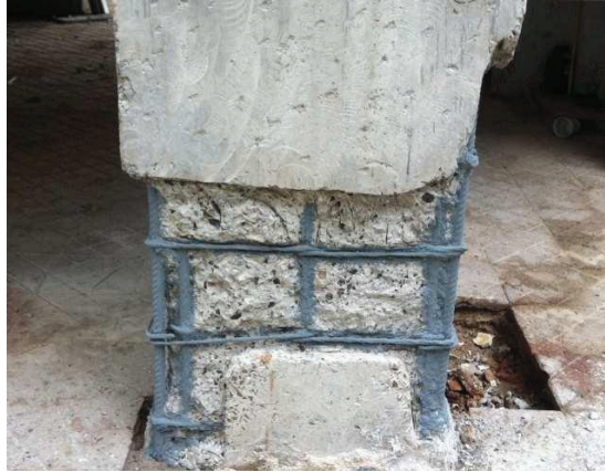
TYPICAL IMAGE OF SURFACE PREPARED RCC MEMBER
